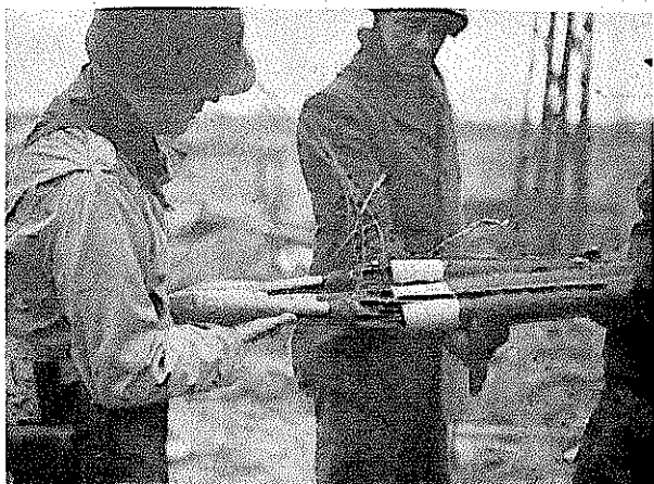
Bazooka shell case slit for wire.
